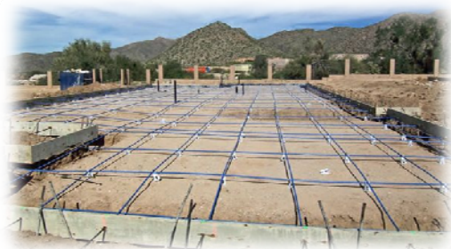
Figure 16: Typical Tendon Layout Photo courtesy of www.tucsonazrealestateblog.com
