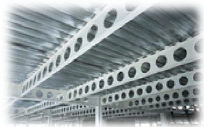
Figure 9: Cellular Beam System Photo courtesy of www.fabsec.co.uk
