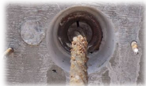
Figure 17: Detail of Tendon Anchor Photo courtesy of www.tucsonazrealestateblog.com
