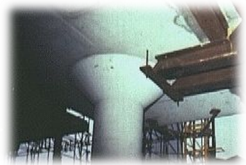
Figure 13: Two-Way Flat Slab with Drop Panels
